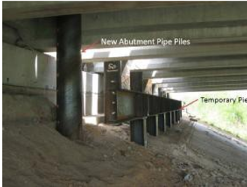
Figure A-18: Repairs and New Foundations (DeStephen, 2015)
